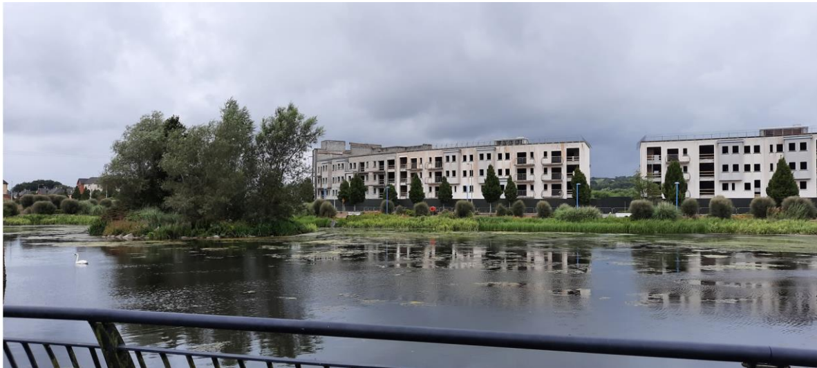
Plate 4-1 Castlelake attenuation pond and adjacent apartments undergoing refurbishment
